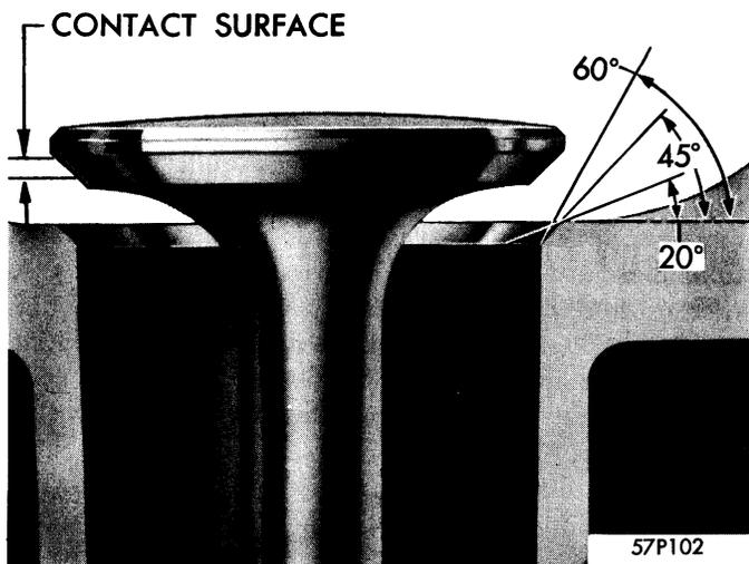
Figure 60—Valve Seat Reconditioning Angles
